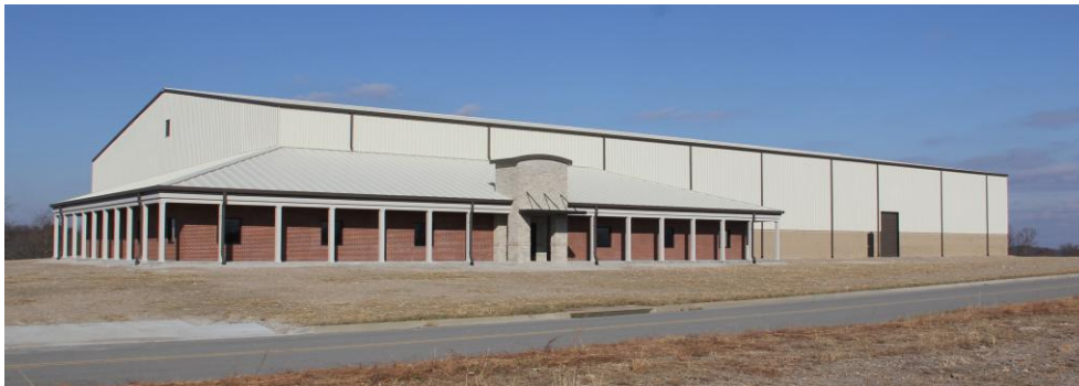
East Kentucky Business Park Spec Building, Martin County
